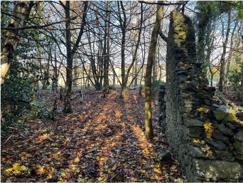
Plate 9: View north along west church gable.
