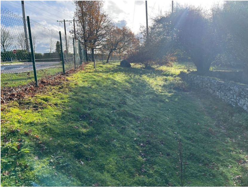
Plate 17: View south along east graveyard wall.
